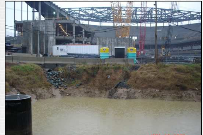
Stormwater Retention Pond
